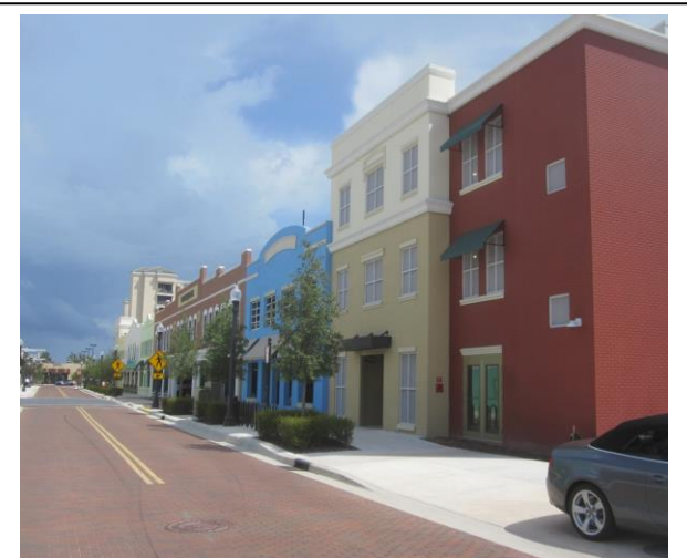
Another parking deck appears as a storefront.
