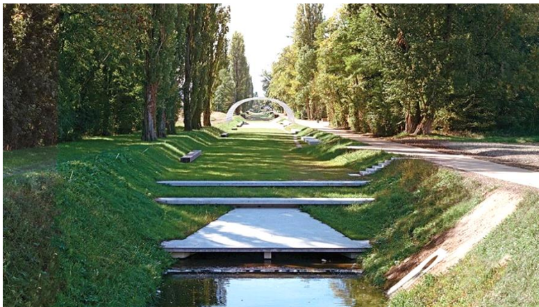
The adjacent drained canal has been transformed into a green space inspired by 19 th century British gardens. Photo by Jasques Bethet.
