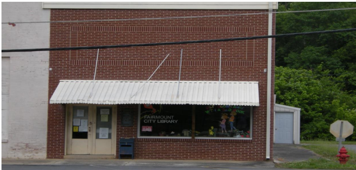
The most rural village center finds a place for the library.
