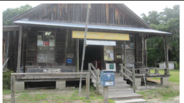
Post offices are found in general stores.
