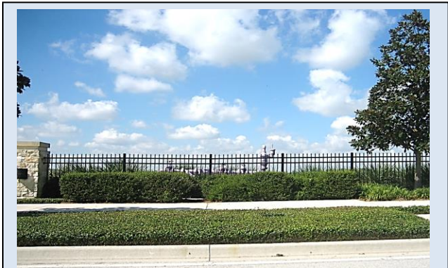
You can barely find the backflow preventor.
