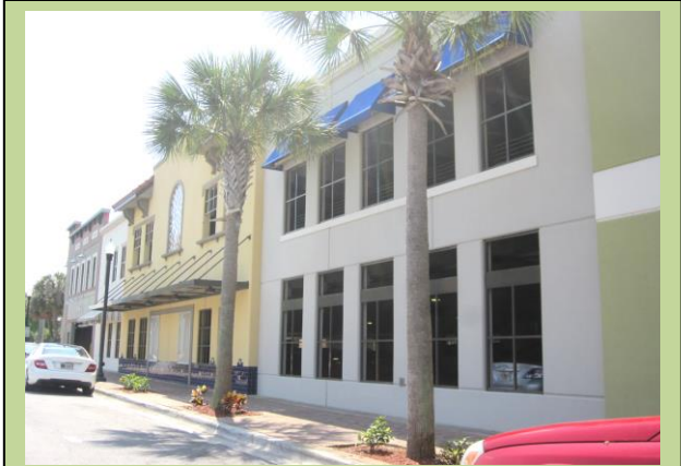
A parking deck disguised as a storefront.
