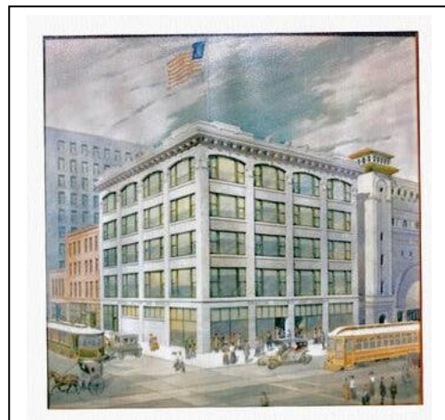
A rendering of the building housing the Denton, Cottier & Daniels music store, designed by Bethune's firm. Completed in 1908, it was one of the first buildings in the country made of steel and fire-resistant concrete slabs. Credit...Kelly Hayes McAlonie
