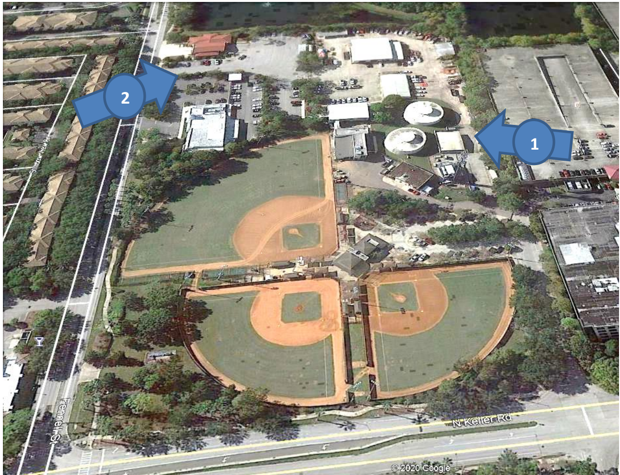
First Station #47 at the top left [1]; public works water plant top right [2] plus ball fields and a concession building. Photo from Google Earth.
