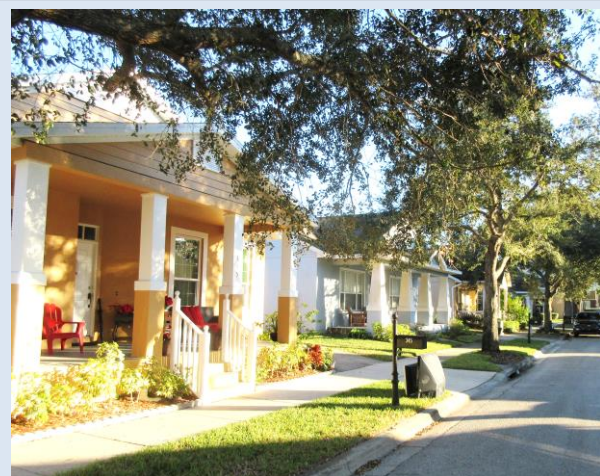
Hampton Park, HOPE VI housing funded by DHUD; A Traditional Neighborhood Development of the Orlando Housing Authority.
