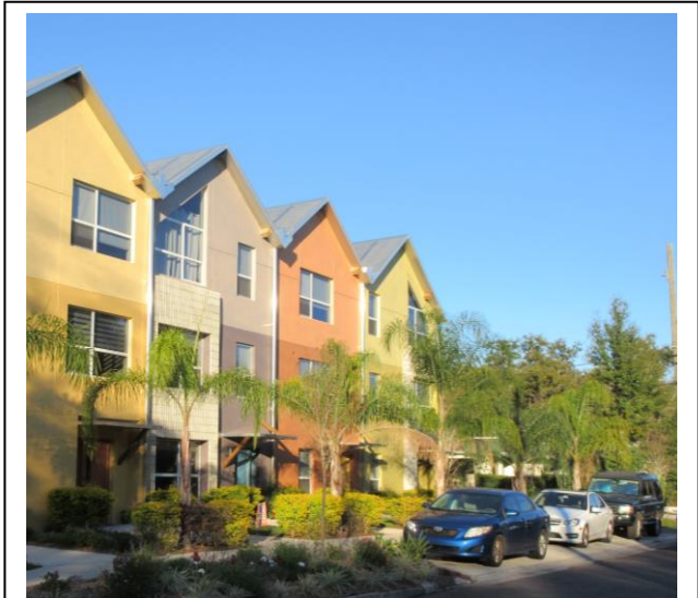
Small complexes of apartments or condos fit nicely on collector streets and corner lots in neighborhoods.
