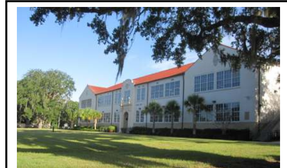
THE PRINCETON SCHOOL BLOCK Princeton Elementary School adjacent to:
